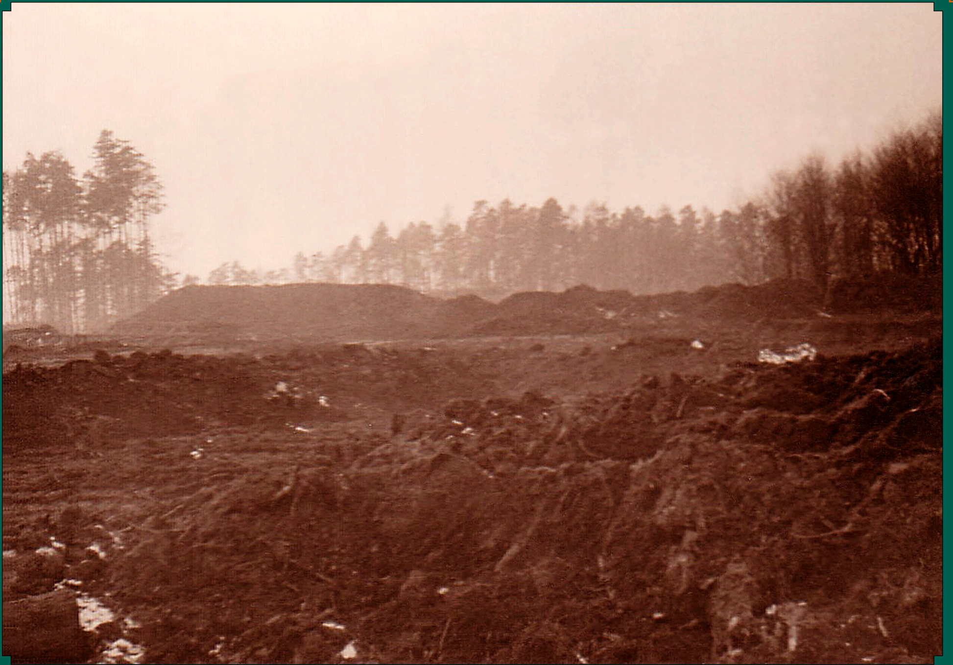
Grading The Launching Area - Spring 1959
