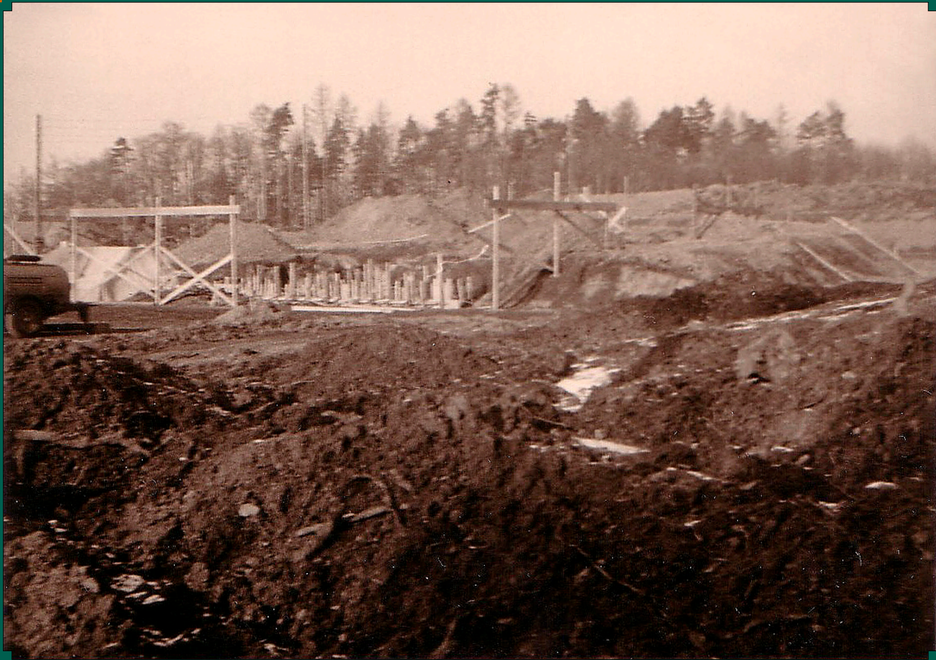
Forming Bravo Section Revetment - Spring 1959
