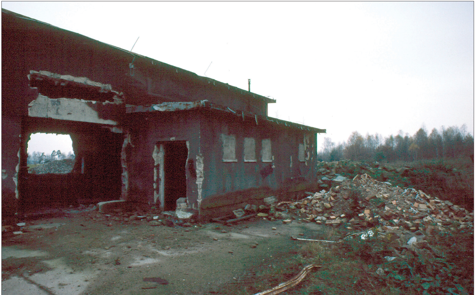
The remains of the Generator building in the Launching Area. It looks like it was built as a cinder block structure, which was probably pretty easy to knock down. Photo: Georg Haeder-1985
