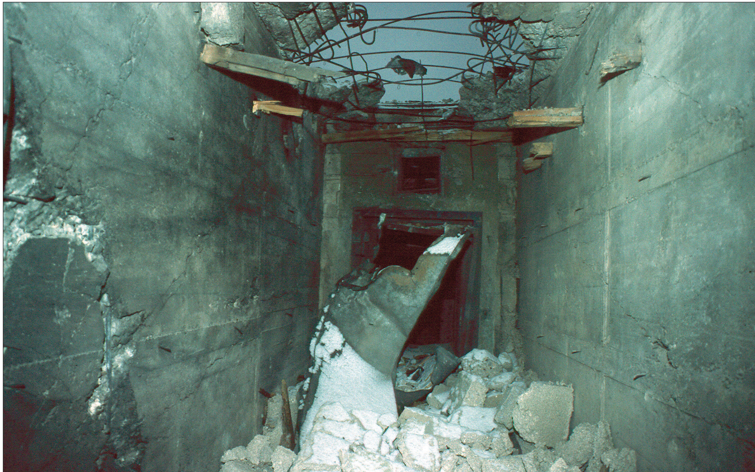
A Section's Revetment passage way to the Section Panel/crew shelter in the process of demolition. Each passage way, front & rear, had two heavy steel doors that sealed the room. Photo: Georg Haeder-1985
