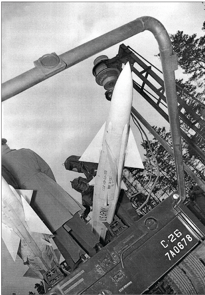
A fueling Demonstration of a Nike Ajax Guided Missile. The wearing of acid resistant suit illustrates the danger
