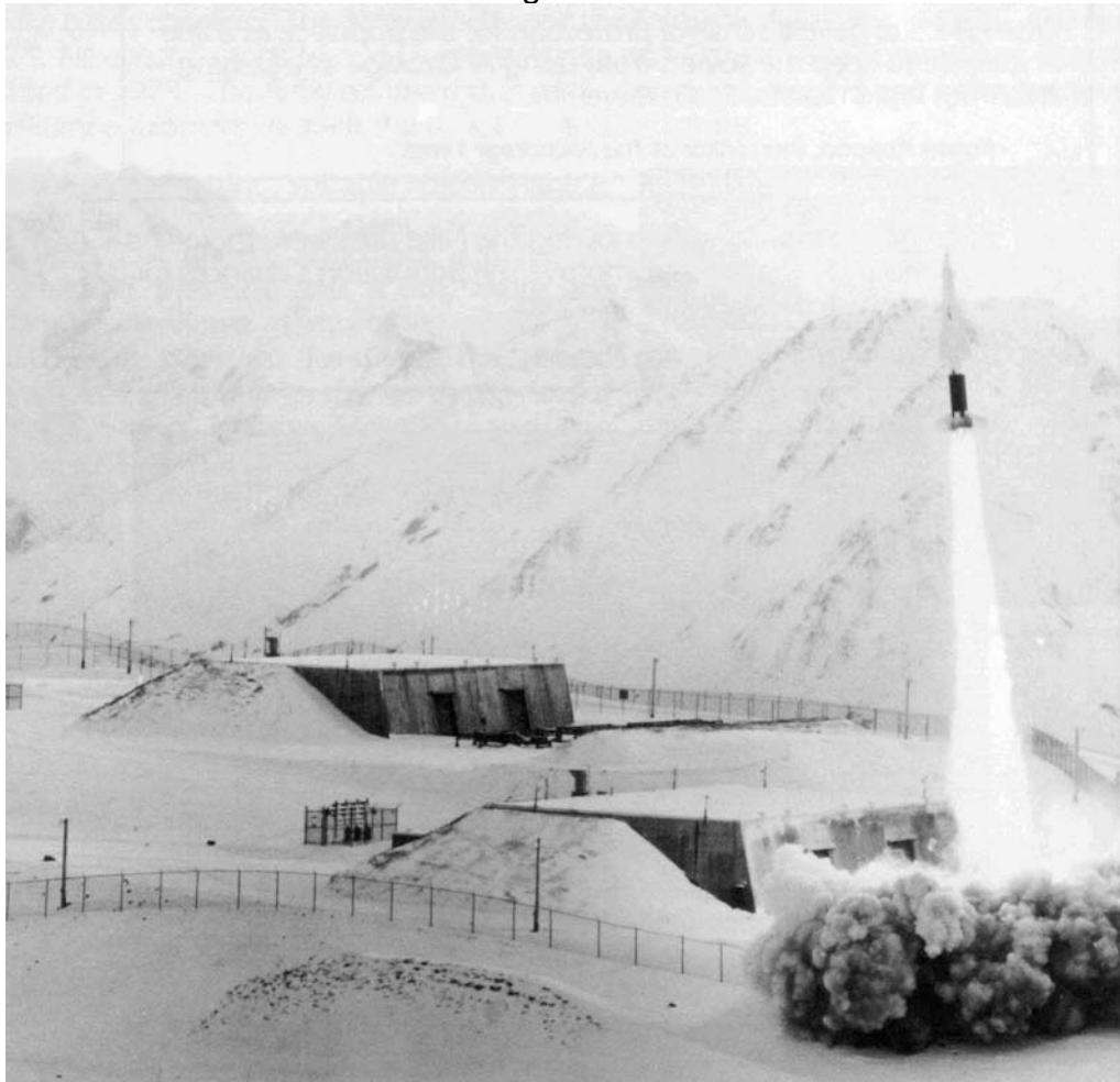
First live fire of a Nike Hercules at Site Summit in Alaska. In the background are the above ground missile storage magazines characteristic of Nike bases in Alaska.
